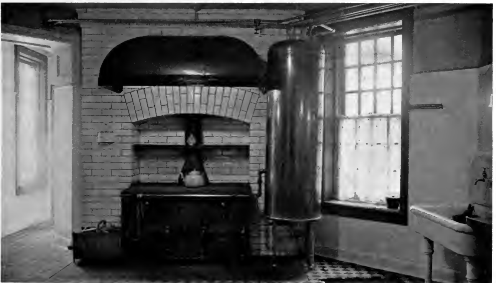
FIG. 8.—KITCHEN IN THE HOUSE OF MR. M. NEWBORG.
